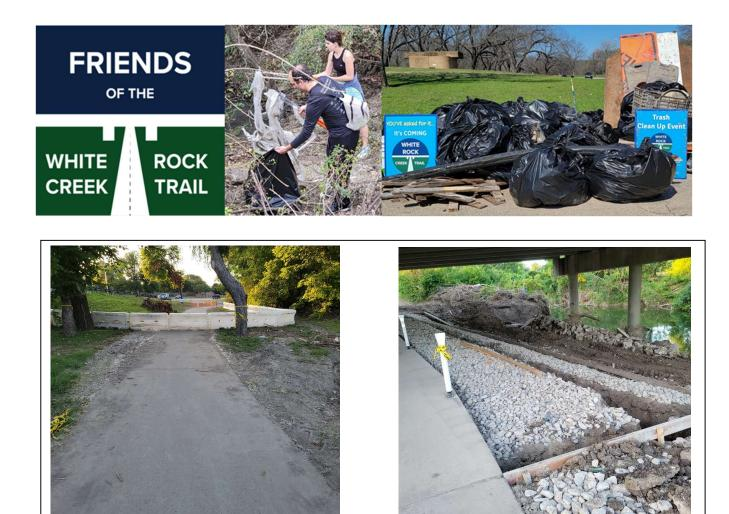
The first two projects dealt with the Royal Ln. underpass, which had gotten dangerous due to multiple high-water events washing out much of the soil under the trail. Barricades had been placed along the side of the trail, but these continued to be moved by high water. The barricades were then used to close the trail. The underpass was rebuilt at 12' wide and a new apron poured. We expect this portion will stay as it is when the whole trail is widened to 12'.
